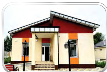
Construction of medical points
