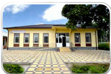
Construction of technological buildings
