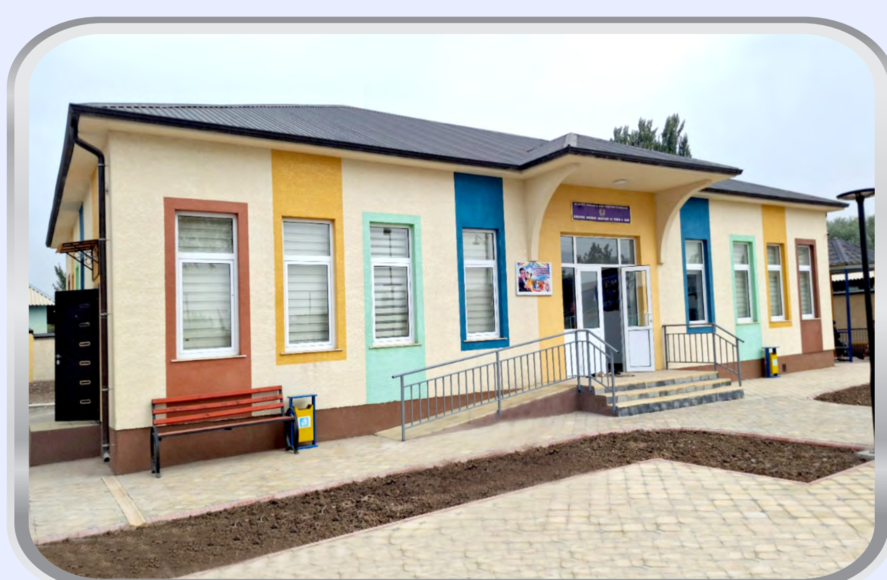
Construction of kindergartens
